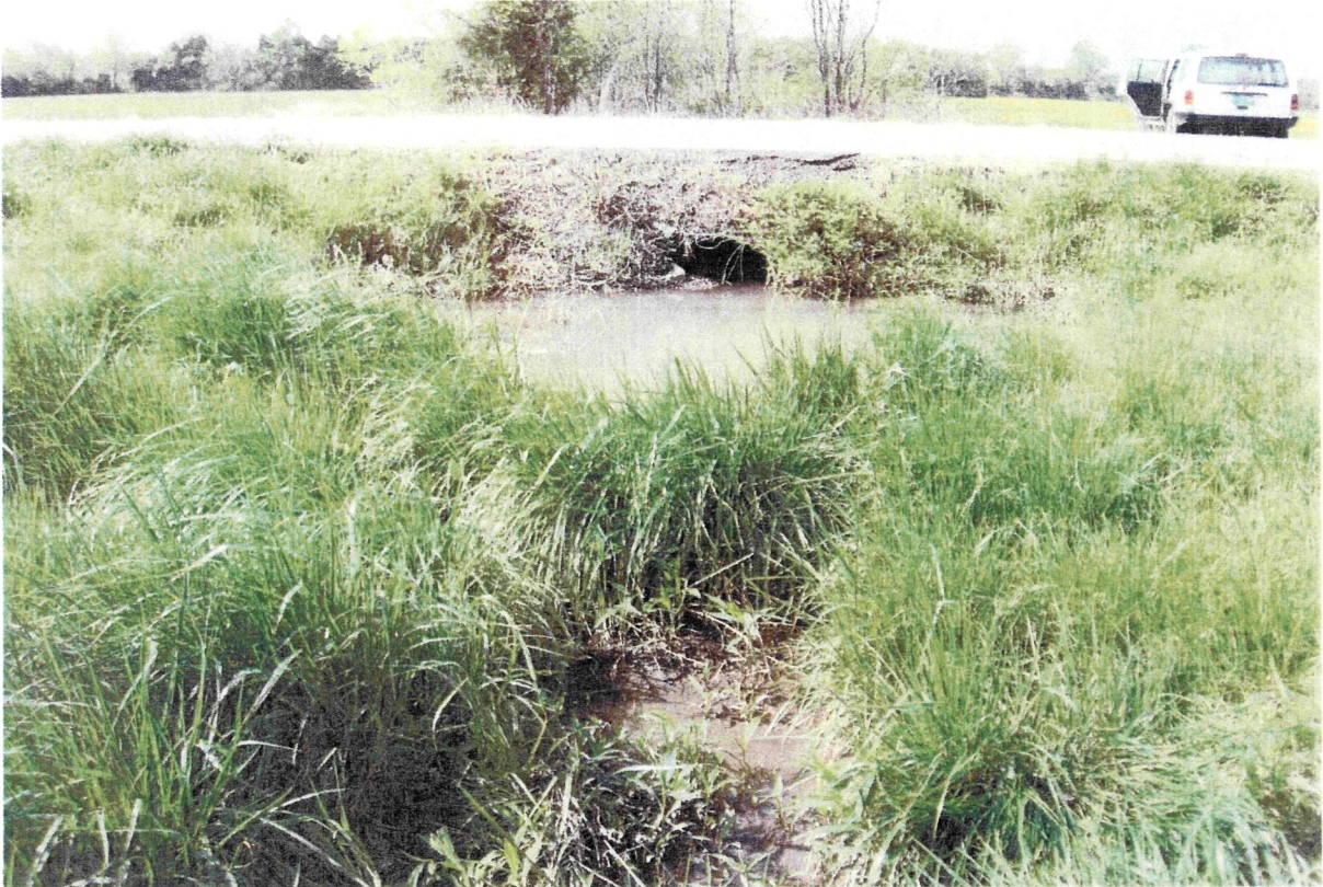
Station 85+33 Lt., Unnamed Tributary to Harpeth River (S-5), photo looking upstream
