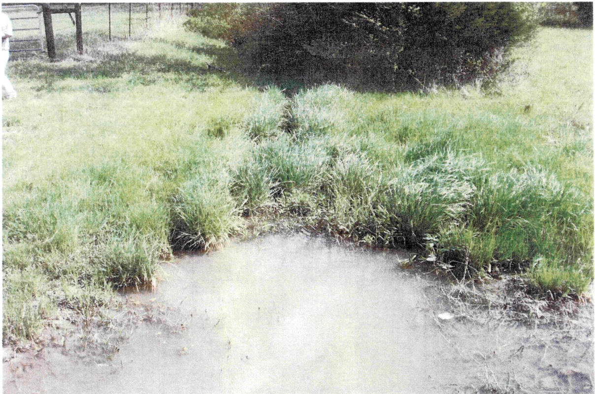
Station 85+33 Lt., Unnamed Tributary to Harpeth River (S-5), photo looking downstream
